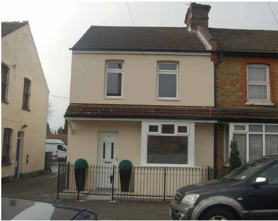
Adjacent terraced house
